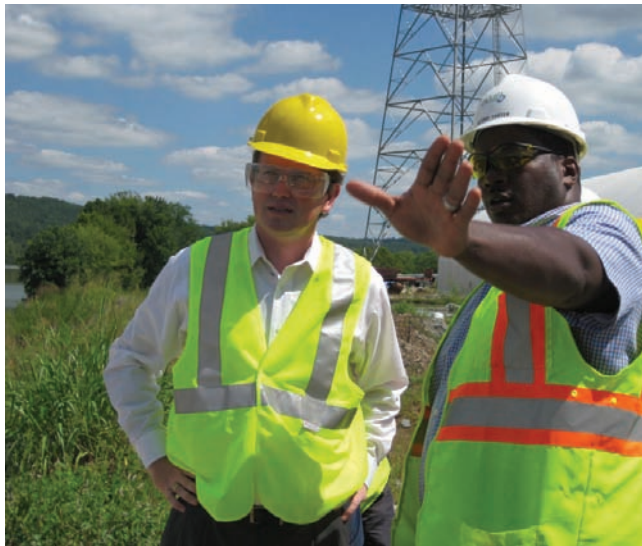
Bishop Carter (right), AMP's Meldahl site manager, discusses construction of the Meldahl hydroelectric facility with Congressman Thomas Massie (R-Kentucky) during a tour on Sept. 4.
